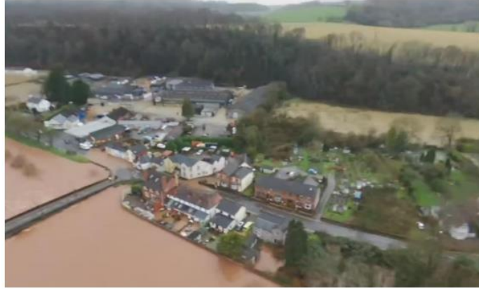
The extent of flooding in Usk in February 2020
